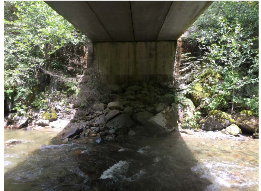
Left Bank Abutment when facing downstream
