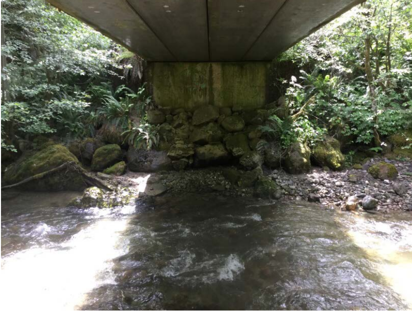
Right Bank Abutment when facing downstream
