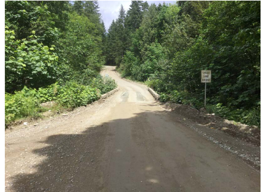
Right Bank Abutment when facing downstream
